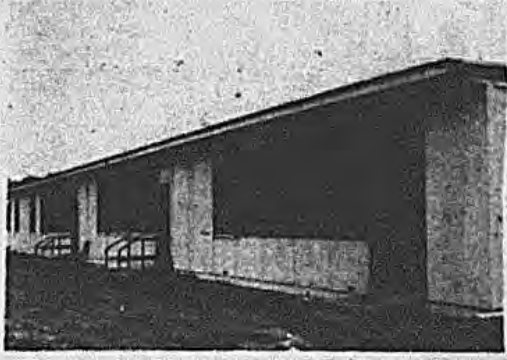
The north wing of the Junior High "temporaries" awaiting the bulldozer last week. Window and door glass was already removed to safeguard and facilitate the demolition. Teachers and classes had easy fire escape drills from these rooms. (Photo by Ed Bady, Hicksville Gregory Museum)
